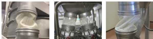
Installation gap too small
