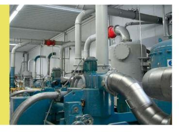
JACOB pipework systems can also be used to convey and extract products in low-pressure applications.
